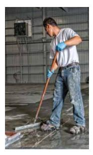
Once the condition of the floor and environment are properly diagnosed and any mitigation steps taken, the next step is surface preparation. The surface of a concrete floor is prepared to increase the porosity, profile and surface area so that the new coating can penetrate, bond and effectively adhere to the concrete. Achieving a rough sandpaper-like profile is ideal. Surface preparation is always best accomplished with these three elements:
